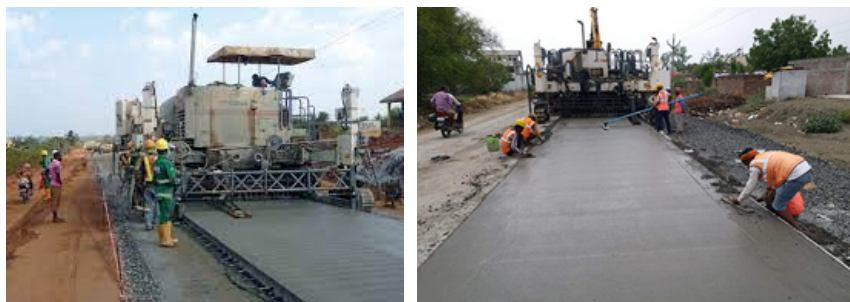
FIGURE 5: CRCP (ADOPTED FROM WWW.RACHANAINFRA.COM AND WWW.WORLDBUILDINGS.COM )
