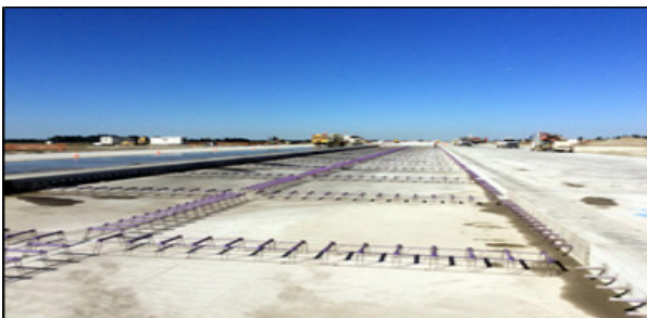
FIGURE 3: REINFORCED CONCRETE PAVEMENT WITH JOINTS. (ADOPTED FROM
