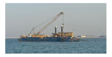
The Pilot hole was drilled from HDD equipment to a designated "exit" point offshore as previously highlighted. HDD equipment is placed on a drilling barge specifically geared with anchor line and SPUDs.
