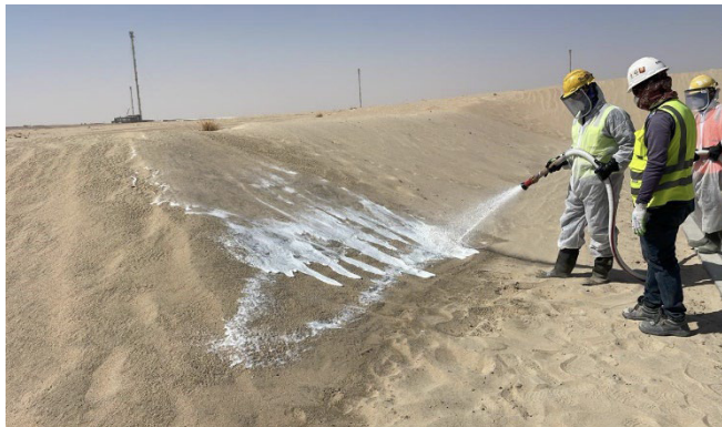
Polymer Spray Application on slopes
