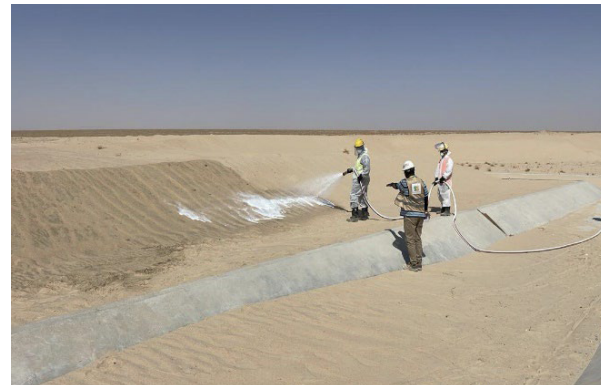
Polymer Spray Application on slopes
