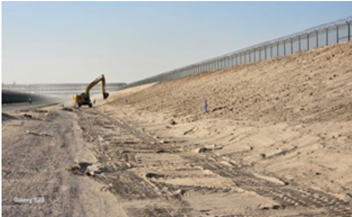
Slope Preparation in East side of Flare Area – for Polymer Spray
