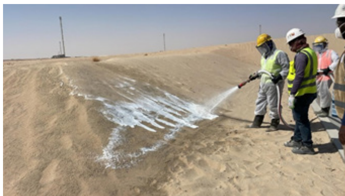
Polymer Spray Application on slopes
